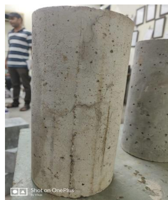
Fig. 9. Surface texture of concrete cylinder after exposure to 600°C for 1 hour duration
