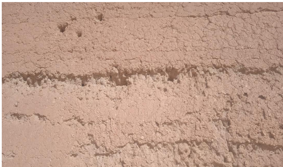
figure 04: The image illustrates the impact of wind on the northern wall of Kasr Melouka Source: The researcher.
