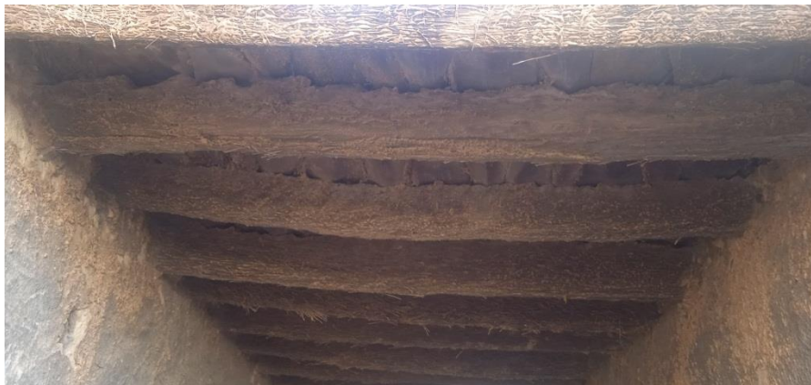
figure 02: The image illustrates the technique of roofing with palm wood.
