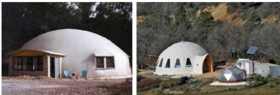
Fig. 2. Curved houses for single dwelling (Courtesy: Ferrocement Society of India)
